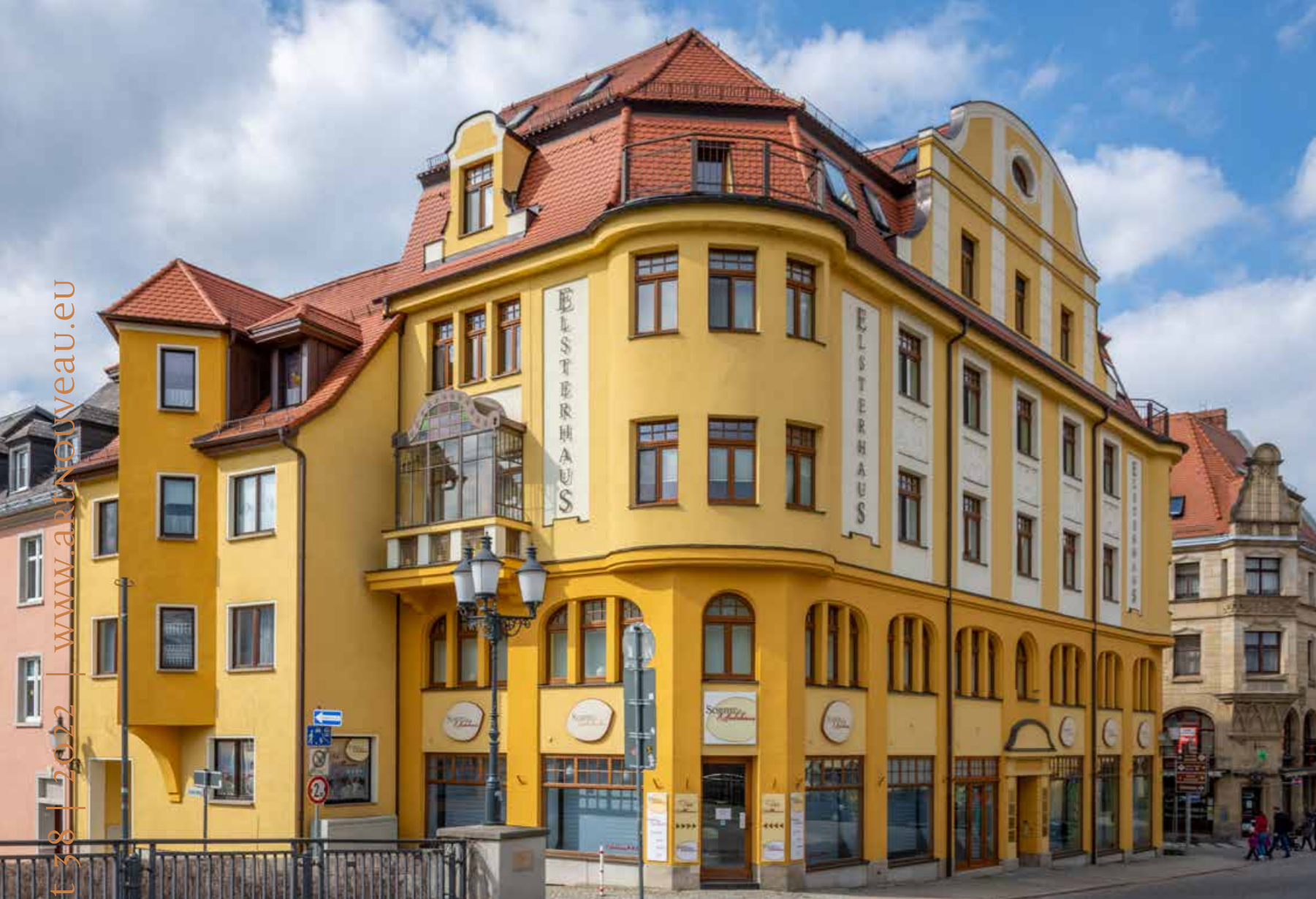
The building at Brückenstraße 3-5. Although planned as a typical department store by Moritz Golle in 1911, it had both residential and commercial uses L'edifici ubicat als números 3 i 5 de Brückenstraße va ser dissenyat com uns grans magatzems per l'arquitecte Moritz Golle el 1911, però va tenir un ús residencial i comercial
